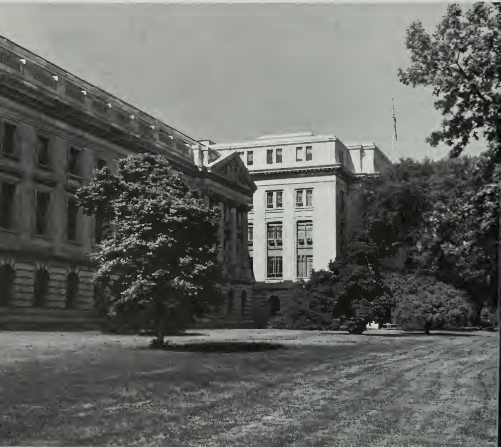
The Administration Building and part of the east wing.
